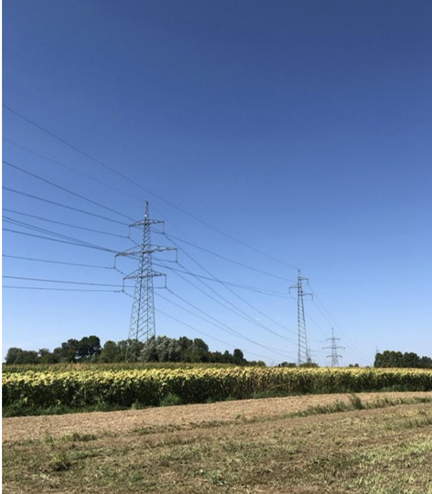
Figure 22. Existing 400 kV line 2xOHL 400 kV Žerjavinec-Heviz
